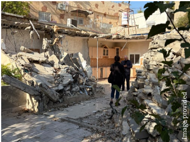
Demolition witnessed by an EA in Silwan.
