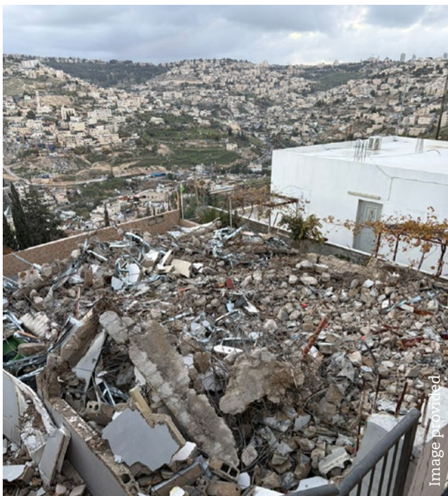
Demolition in Jabel Makaber.
