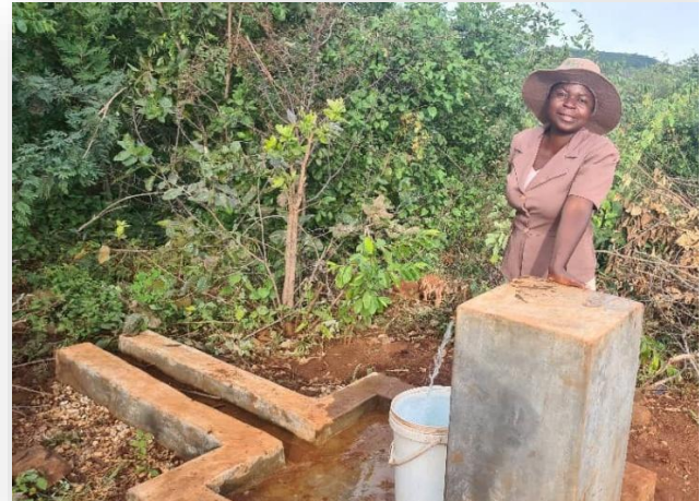
Figure 21: Some taps were left leaking and with no handles, while other points are well managed
